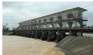
Water intake facility, Da Nang, Vietnam
